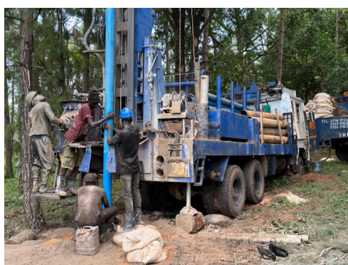
Above, bore hole drilling at Acheru.
