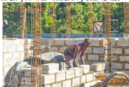
Above, the new stored office building which will house most of the departmental offices and the International office .
