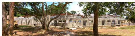
Above, the new primary school building block in Mukono.
