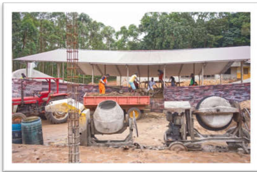
Above, our youth constructing the ark.
